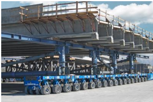
BRIDGE AND TUNNEL CONSTRUCTION
